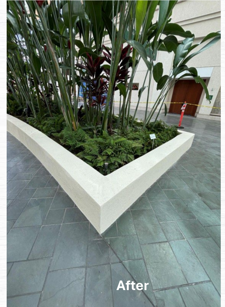
3rd Floor Center Concourse planters spalling repair and resurfacing.
