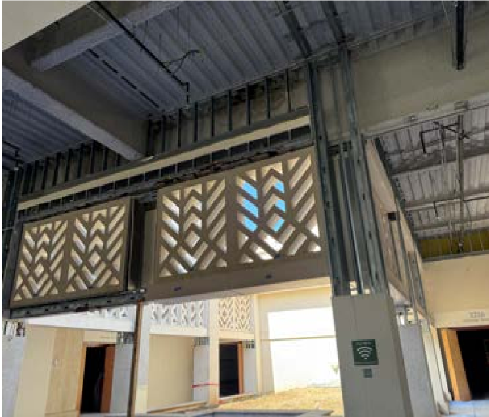
Level 3 – Demolition Continues
