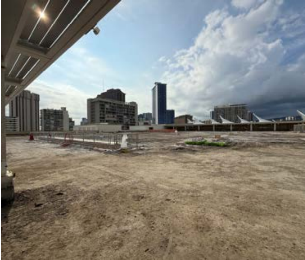
Level 4 – Overall Demolition of Rooftop Finishes and Topping Slab Complete
