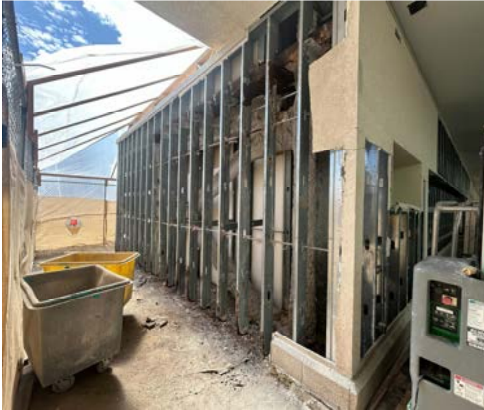
Level 4 – Bathrooms Perimeter Wall Demolition in Progress
