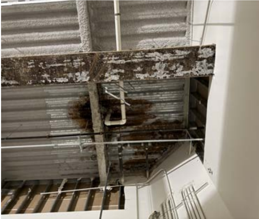
Level 3 – Fireproofing Removal in Progress in Preparation for Structural Repairs
