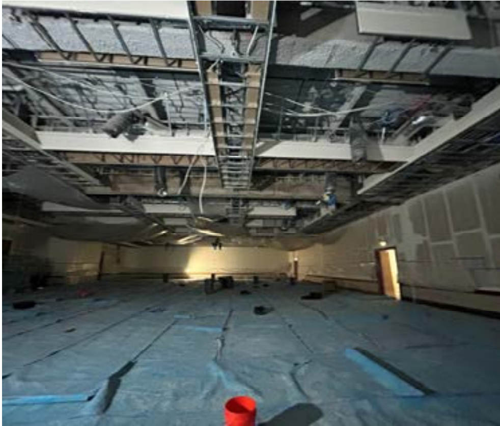
Level 3 - Meeting Rooms Ceiling Removal Complete and Steel Deck Fireproofing Removal in Progress
