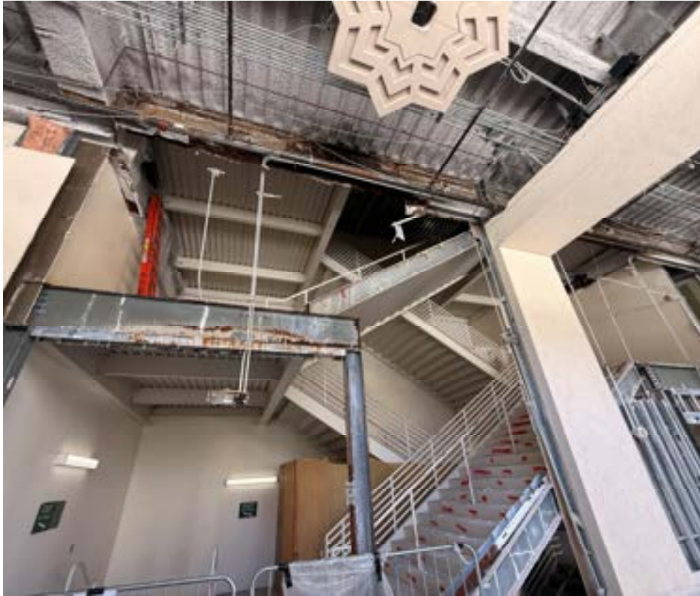
Level 3 – Stair 5 Selective Demolition in Progress and Structural Fireproofing Removal in Progress
