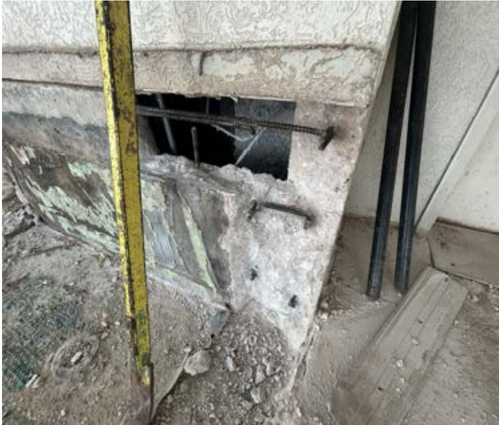
Level 4 – Selective Demolition in Progress – General Structural Repairs - Spalling
